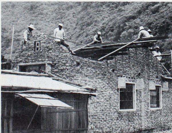
"New brick houses in various stages of construction. . . ."
